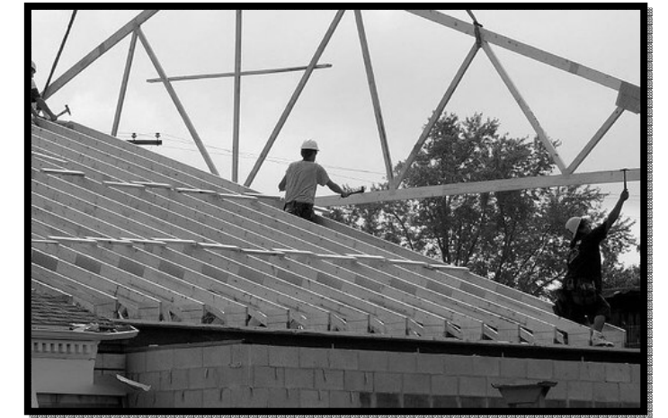
Up go the roof trusses
